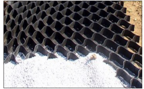
Cellular confinement panels being backfilled with gravel
